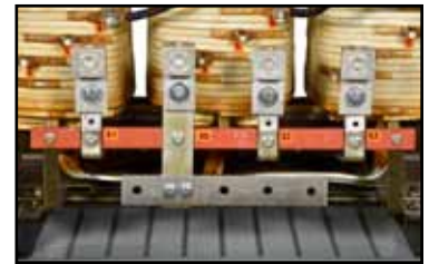
Expanded neutral bar for multiple customer connections
